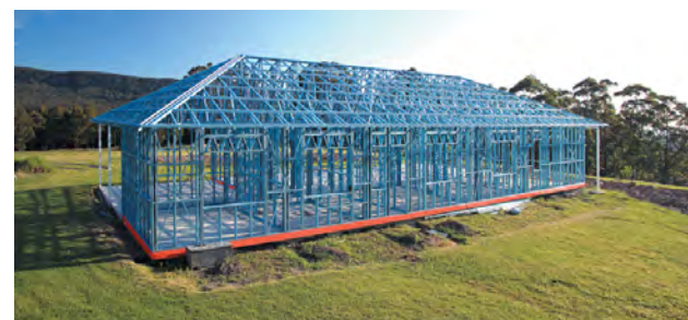
Example of house built using non-combustible framing material (steel frame). Source: KNK Builders
