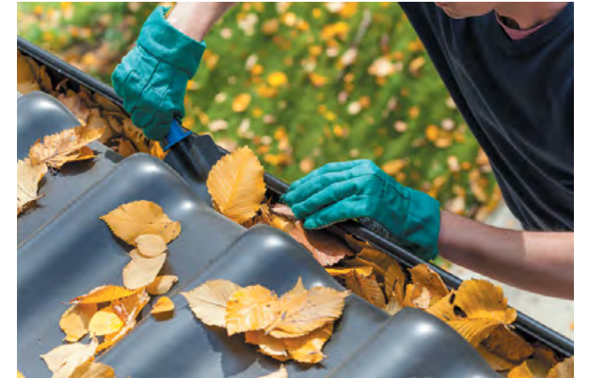
Regularly clean debris from your gutters.
