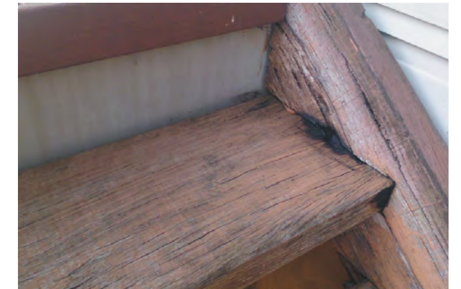
Ember attack in re-entrant corners. Source: CSIRO
