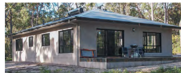
Example of bushfire resistant building. Source: Paul Whittington
