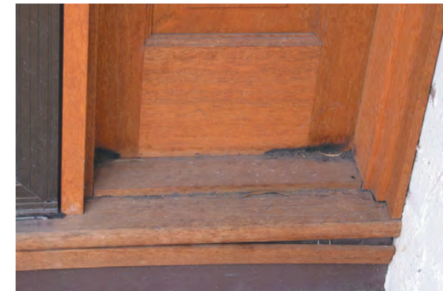
Embers attack in re-entrant corners. Source: CSIRO
