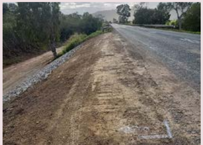
Bruce Highway (Mackay–Proserpine) – completed batter repairs (July 2023)
