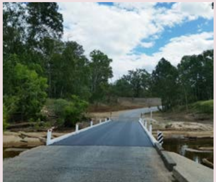
Laura River bridge – completed bridge repairs (July 2023)
