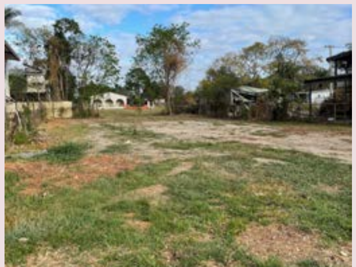
9 Enid Street demolition complete
