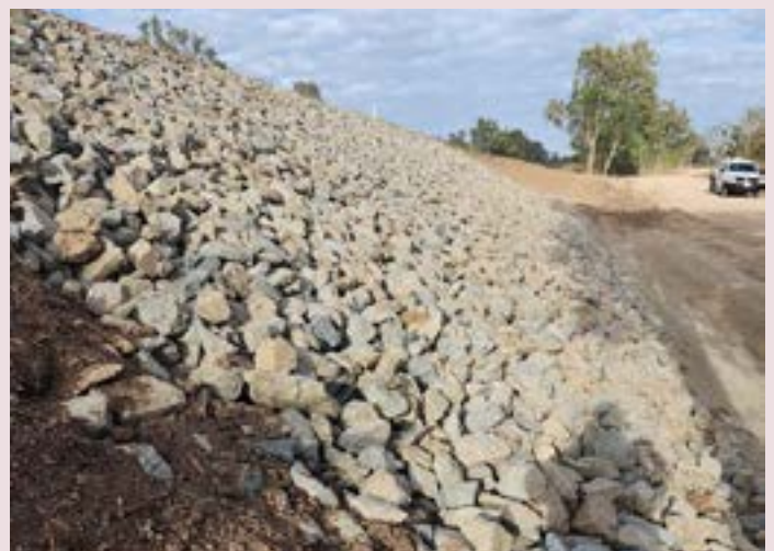
Bruce Highway (Mackay–Proserpine) – completed batter repairs (July 2023)
