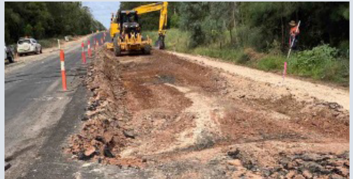
Moonie Highway (Dalby–St George) – floodway reconstruction works (January 2023)
