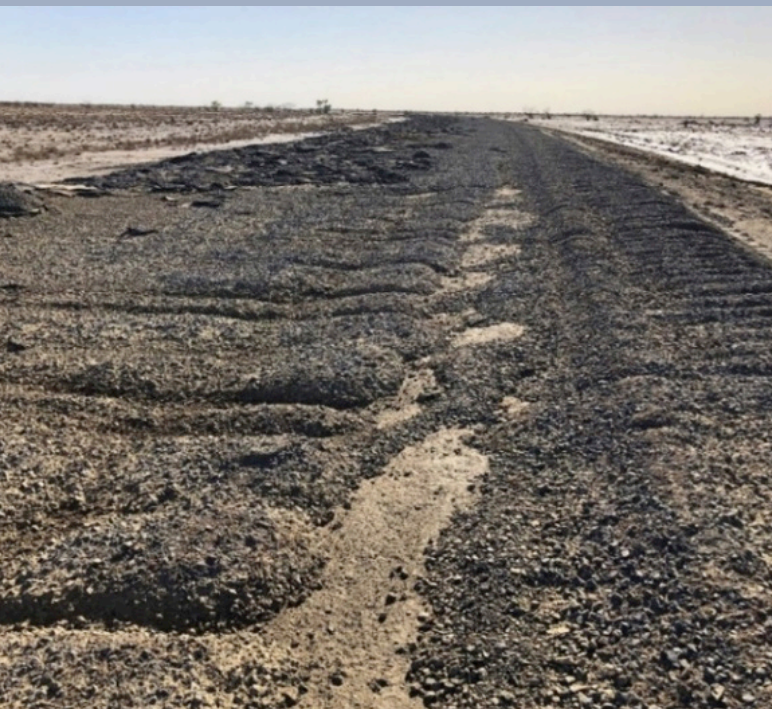
Image: damage from the Monsoon Trough event.
