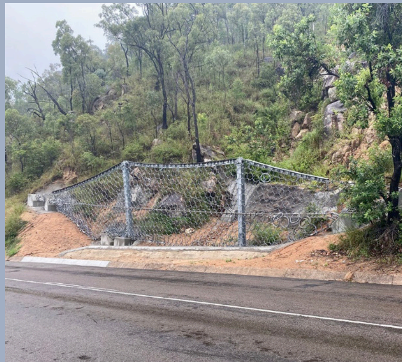
Image: completed repairs.
