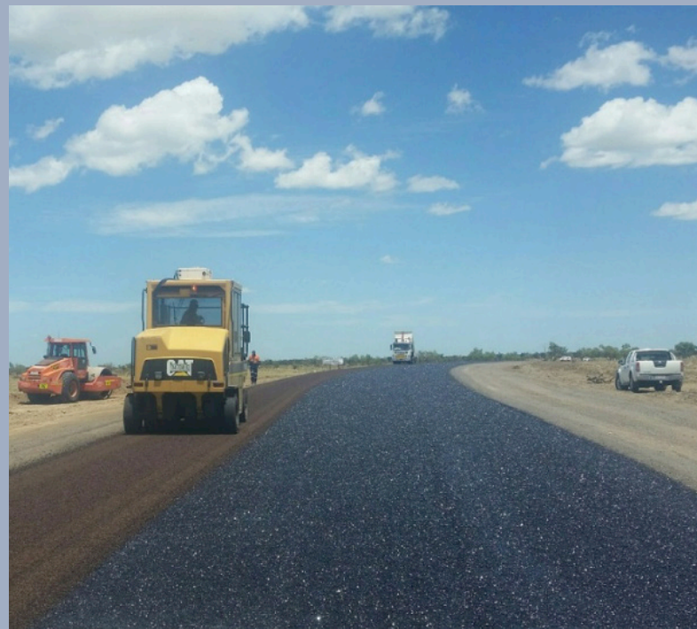
Image: emergency works.
