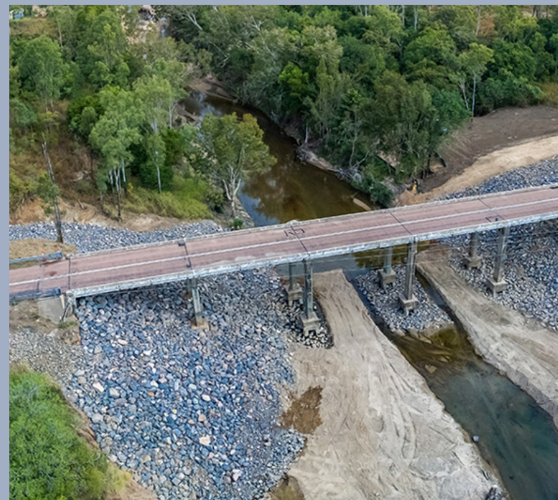
Image: completed repairs.
