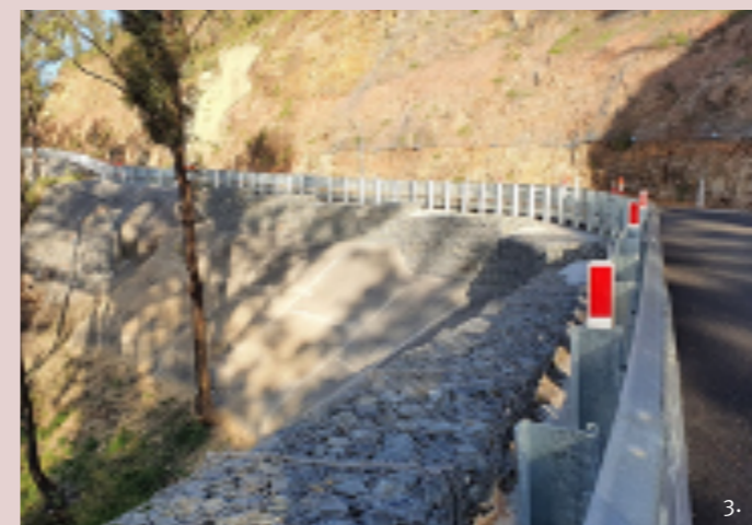
Images: (1.) Binna Burra Road – rock descaling with long reach excavator (2.) Binna Burra Road – drape mesh and rock gabions (3.) Binna Burra Road – rock gabions and drape mesh (4.) Binna Burra Road – workers abseiling down steep slopes to install soil nails.
