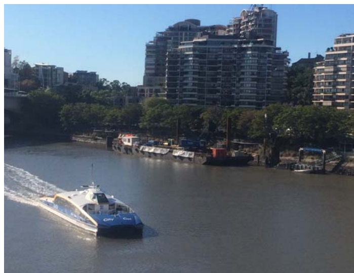
Piling works underway on Maritime Museum ferry terminal - October 2014
