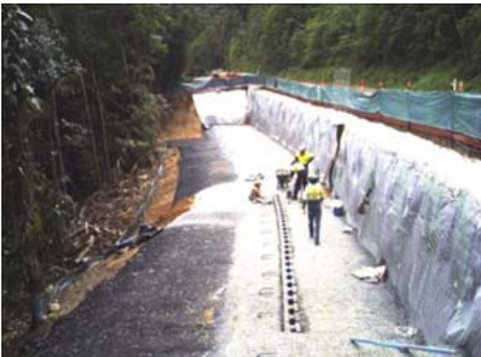
Yarrabah Range Road during reconstruction and betterment works
