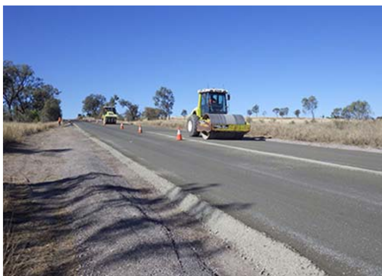
Above: overlay works on the Dawson Highway
