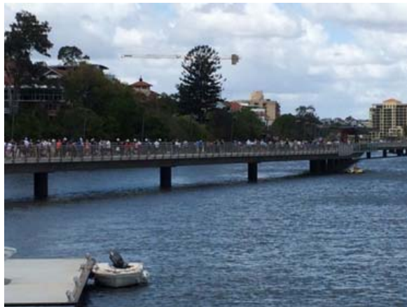
The damaged Brisbane Riverwalk following the 2011 floods (top), and at its re-opening after completion of reconstruction work on 21 September 2014 (bottom)
