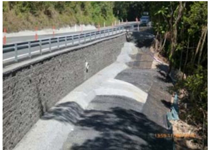
Yarrabah Range Road betterment project following completion—September 2014
