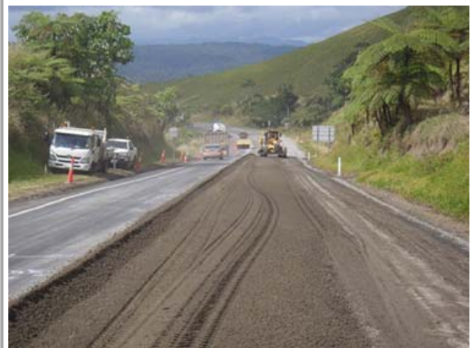
Above: Palmerston Highway – final trim of base
