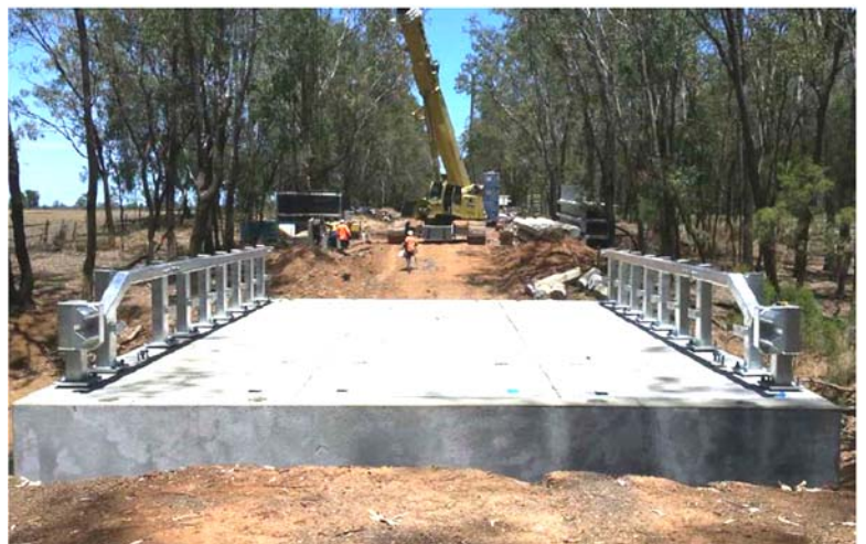
Boolburra Edungalba Road Betterment project under construction - October 2016
