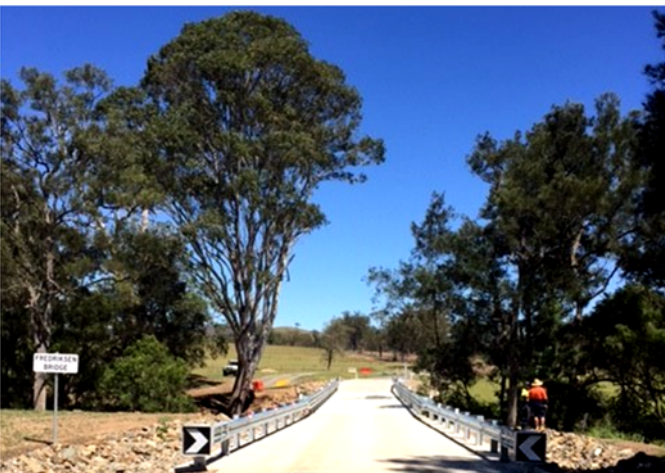
Damage to Monsildale Bridge following Tropical Cyclone Marcia flooding (top); during Betterment works construction (middle) and the completed and re-named Frederickson Bridge (bottom)
