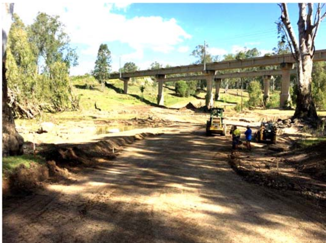
Aroona Road Betterment project under construction - October 2016
