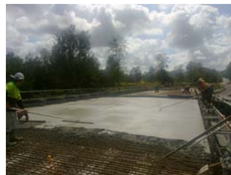
Above: Grigor Bridge reinforcing steel (left), box culverts and embankment works (centre) and first deck concrete pour on 31 October 2013 (right).
