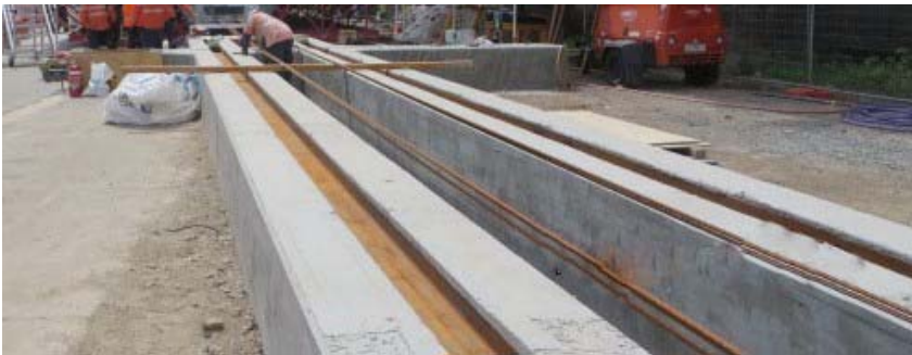
Above: preparing the rail system to move the first pre-cast girder along the Howard Smith Wharve site
