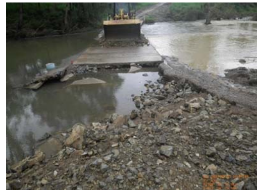
Above: damage to the floodway of Upper Ulam Road, Rockhampton Regional Council
