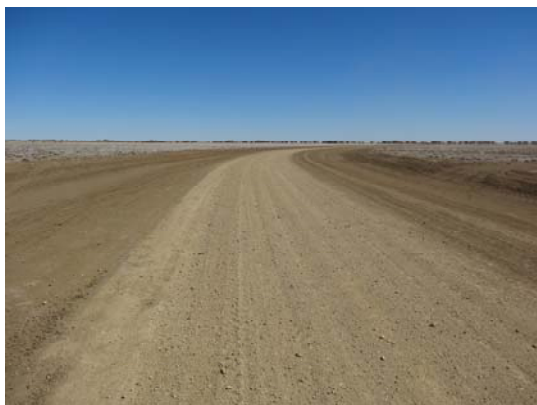
Left: following completion of works, Ardrin Lane, Richmond
