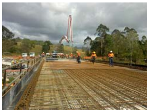
Above: Grigor Bridge reinforcing steel (left), box culverts and embankment works (centre) and first deck concrete pour on 31 October 2013 (right).
