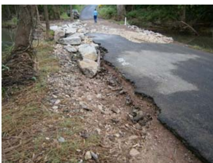
Above: Flood damage to Somerset Regional Council road network— Lake Manchester Road (left); Ted Skinner Crossing (centre); and George Bell Crossing (right)
