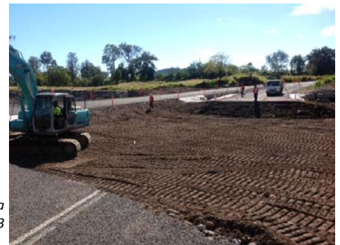
Right: Excavation at Location 1, Mt Sylvania Road, July 2013
