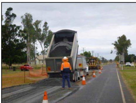
Above: Isis Highway (Biggenden to Coalstoun Lakes) – pavement repairs in progress
