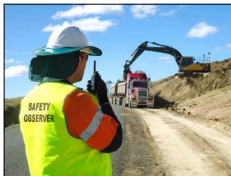
Above: Safety observer for road reconstruction works—Roma-Taroom Road
