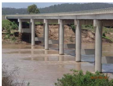
Above: Embankment slip at the Tim Fischer Bridge during Tropical Cyclone Oswald natural disaster event, Bruce Highway, Wide Bay/ Burnett Region
