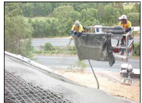
Above: Pacific Highway (Tugun Bypass) - landslip repairs
