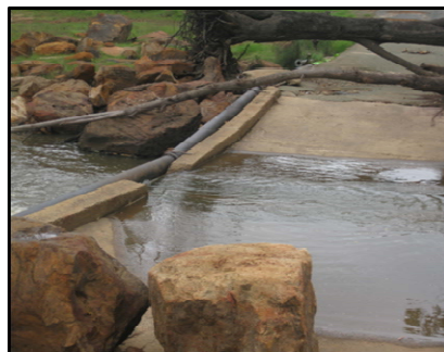
Above: Damage to Mimosa Creek Crossing as a result of flooding in early 2013
