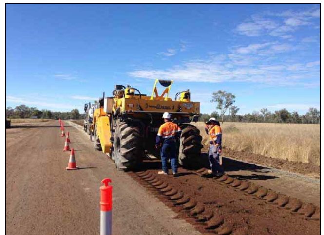
Above: Stabilising works—Dawson Highway (Rolleston to Springsure)
