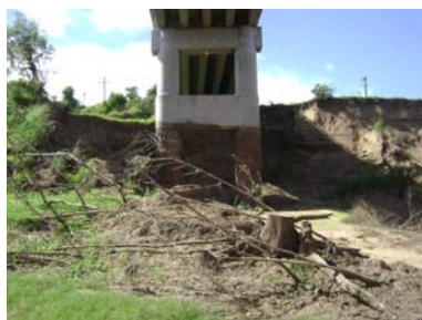
Above: Embankment slip at the Tim Fischer Bridge during Tropical Cyclone Oswald natural disaster event, Bruce Highway, Wide Bay/ Burnett Region
