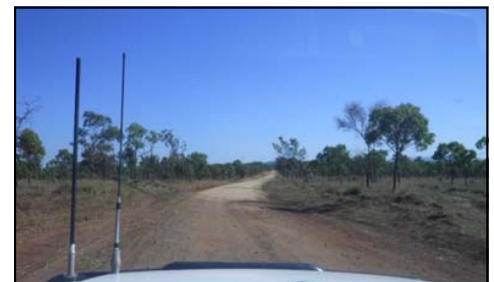
Above: Completed works for the restoration of Dotswood Road.
