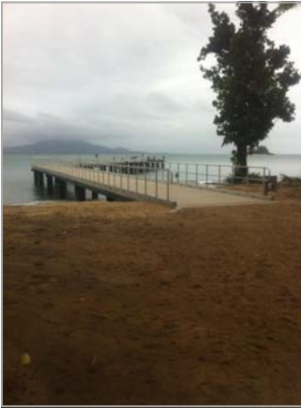
Above: Completed works—Dunk Island jetty.
