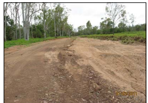
Above and left: Damage to Dotswood Road following heavy rainfall and flooding of March 2012.
