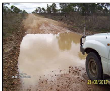
Above and left: Damage to Dotswood Road following heavy rainfall and flooding of March 2012.
