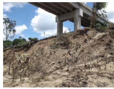
Above: Embankment slip at the Tim Fischer Bridge during Tropical Cyclone Oswald natural disaster event, Bruce Highway, Wide Bay/ Burnett Region
