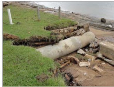
Above : Damage to sections of Palm Island the seawall following Tropical Cyclone Yasi.
