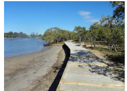
Above: damage (top) and post-completion (bottom) Berree-Badalla boardwalk
