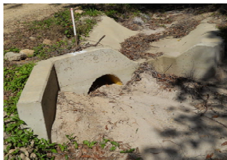
Left: damage to Wunga Road, Yarrabah as a result of Tropical Cyclone Yasi
