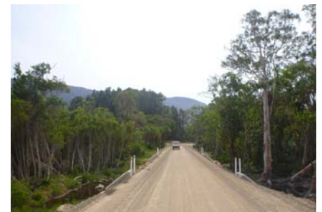
Above: completed works Wunga Road, Yarrabah
