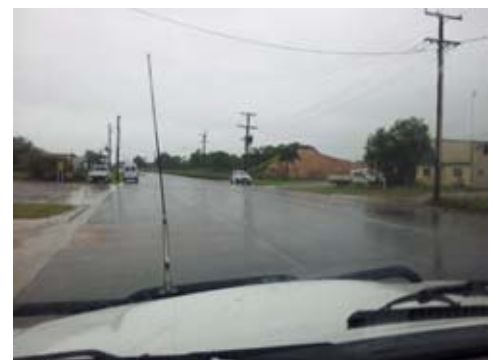
Above: Ingham industrial precinct under flood (top) and following completion of works - Challands Street, Ingham (bottom)
