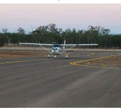
PROJECT FINISHED: Mundubbera Aerodrome is back in action.
