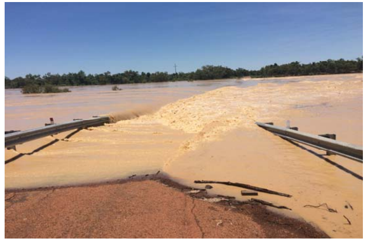
Floodwaters submerge the Little Bynoe Crossing—January 2016
