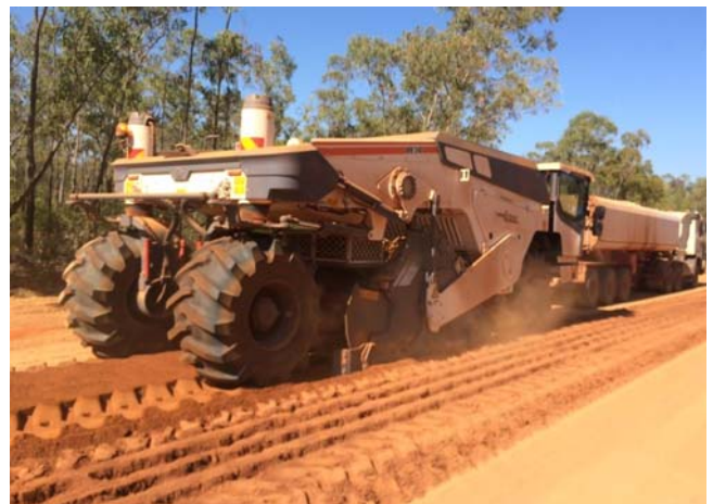
Mornington Island road works
