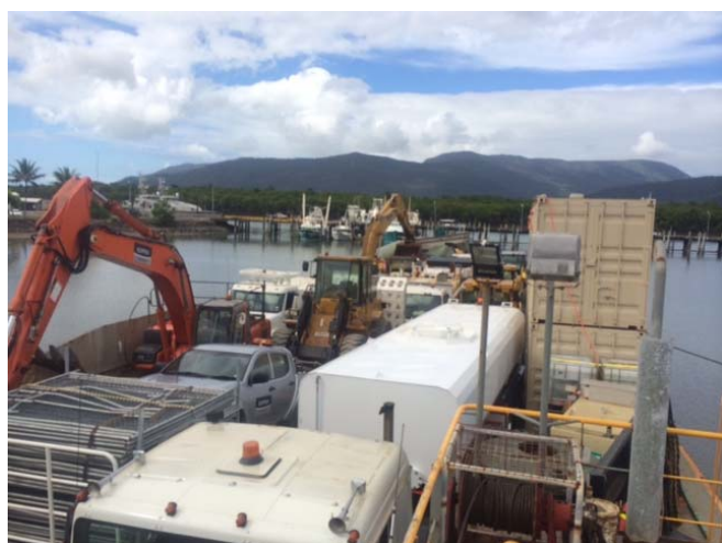
Construction equipment being barged to Mornington Island
