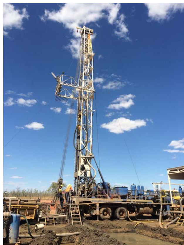
Drilling for bore water, Carpentaria, October 2015
