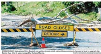
ROAD CLOSED. The Shire of Livingstone Shire Council are waiting on a sign-off against the government to fund a upgrade. The Shire may also be used designed by Cyclone Marcia. PHOTO: CHRIS ISON FOR QSLDRECONSTRUCTION.ORG
