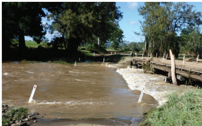
Damage to the existing Jerome Bridge following STC Debbie
