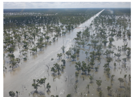
STC Nora dumped rain on already flooded catchments in Far North Queensland, turning Coralie Road in Croydon Shire into a waterway
