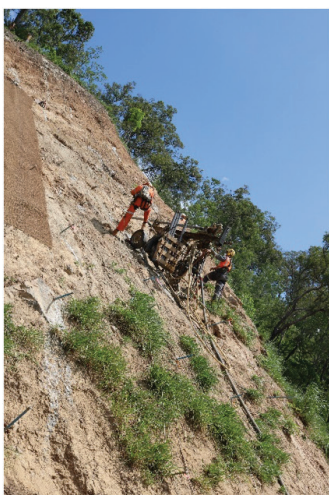
Above: Drilling for the soil nails at the main landslip site, Marlborough–Sarina Road
