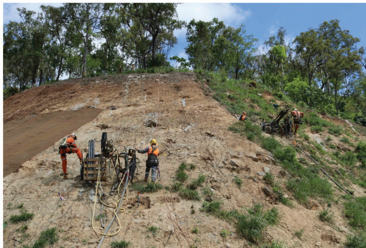
Above: Drilling for the soil nails at the main landslip site, Marlborough–Sarina Road
